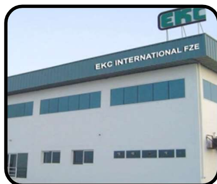
Plant II – Dubai
