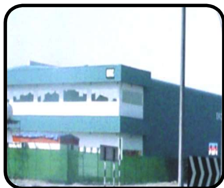
Plant I – Dubai
