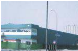
PLANT I, DUBAI
