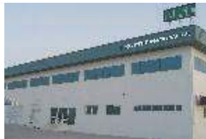
PLANT II, DUBAI
